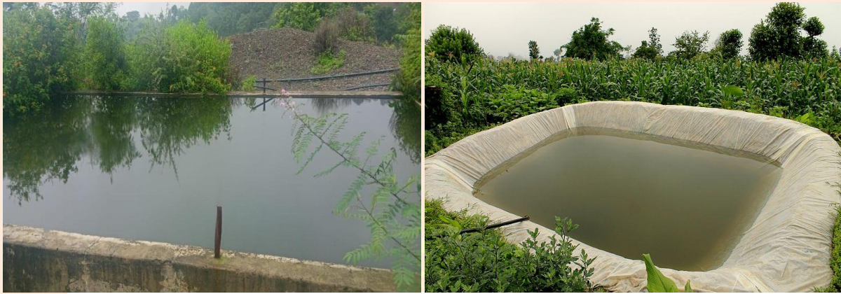
Fig. 1: Rainwater harvesting ponds A) Cemented Pond (B) Plastic pond
